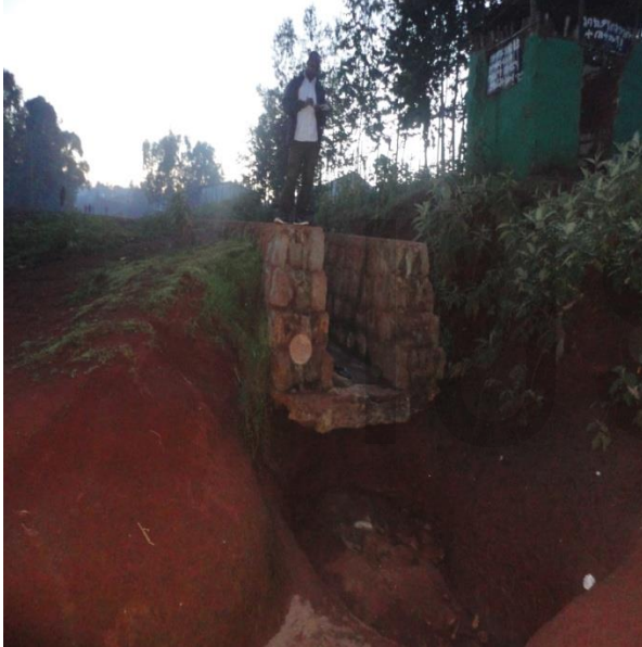
Figure 4.8: Shows unprotected outlet of the drainage canals impact on natural environment (causes soil erosion, stream pollution and its structural failures). (Source: Field survey on July, 2014)
