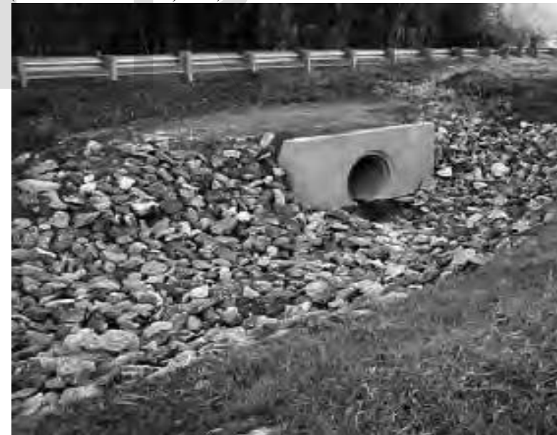
Figure 2.2: Riprap Outlet Protection of Pipe Drains
