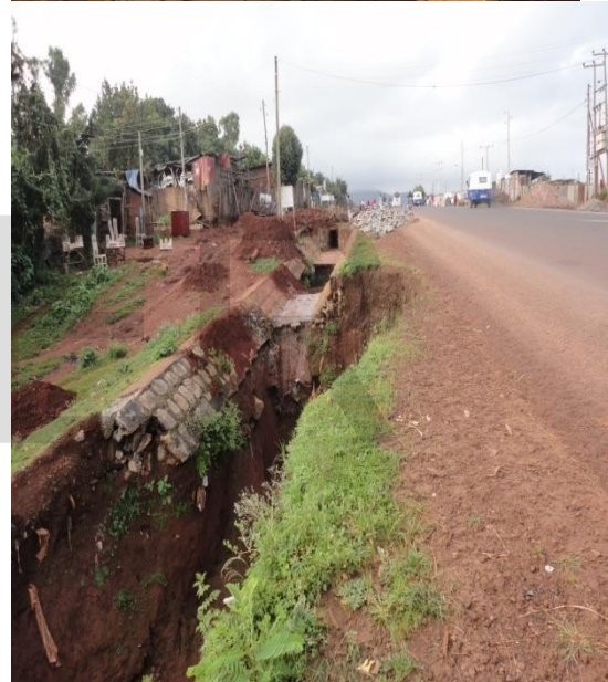
Figure: 4.3 Inadequate Road drains and Ditch Erosion. (Source: Field survey on June, 2014)
