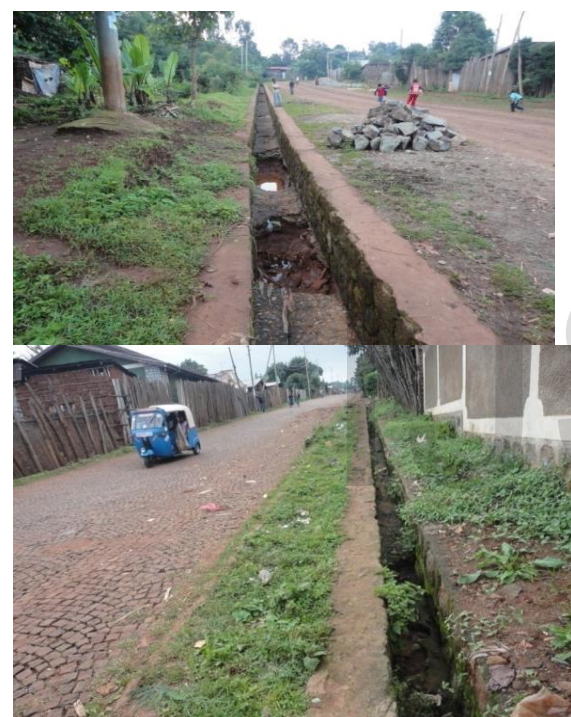
Figure4.6: Road ditch erosion because of steep slope and flow over permissible velocity. (Source: Own Field survey on July, 2014)
