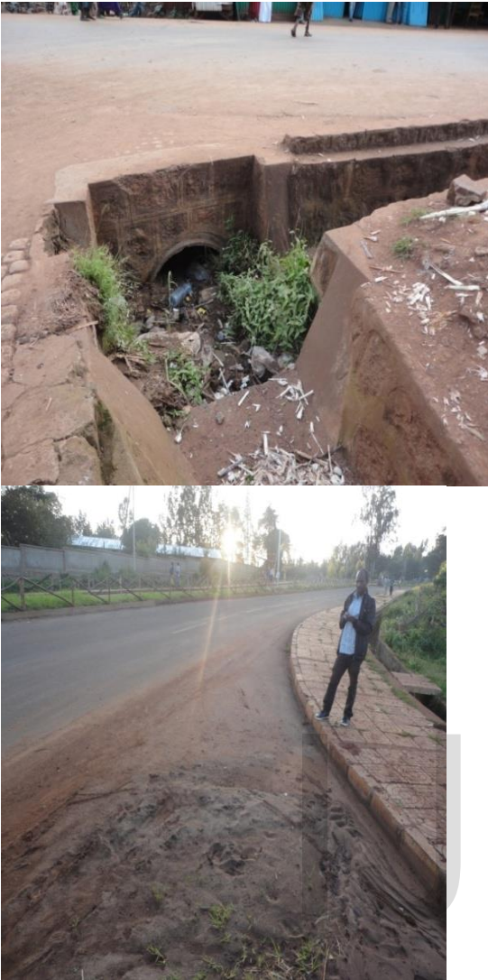
Figure: 4.2. The storm drains are blocked by solid wastes and silt. (Source: Field survey on June, 2014)
