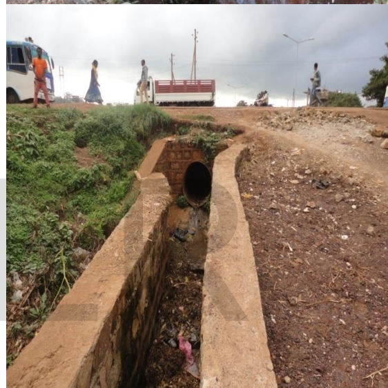
Figure 4.7: Cross drainage structures impacts on the environment (downstream gully formation and solid wastes accumulation). (Source: Field survey on July, 2014)
